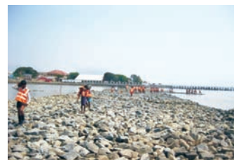
Construction of Rubble-dyke in progress at Sittwe
